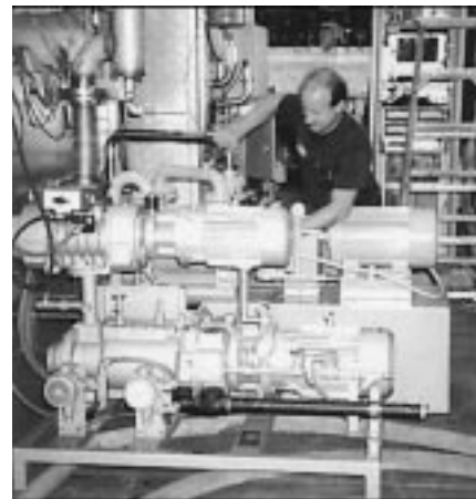
Chris Terwilliger, of the Lyo Renewal Division, monitoring the COBRA/blower system
